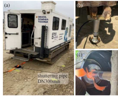
Figure 4. Performing field tests, CPT truck arranged over the artificial test pit (a), preliminary load tests using a hydraulic jack and an excavator as counterweight (b), CPT-piston used for load application during the test (c).
