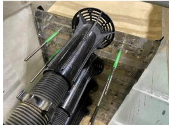
Figure 5. Support in front of facing panels and insertion of soil nails.
