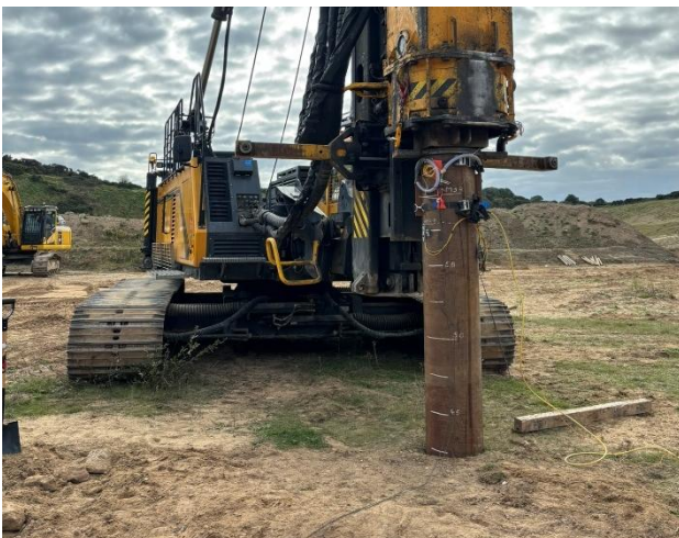
Figure 3. Impact driving of Pile AM345
