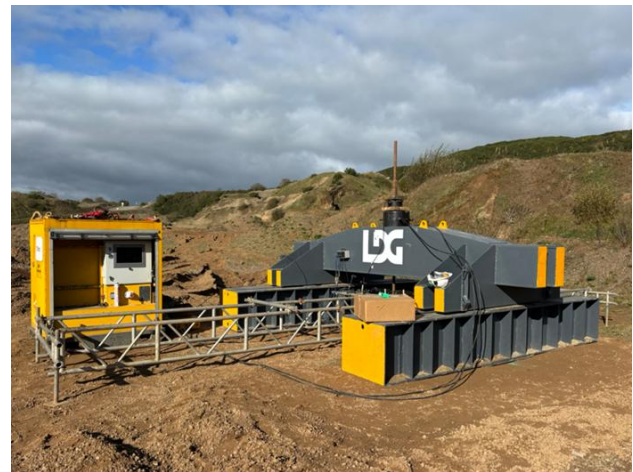
Figure 4. Tension load test setup
