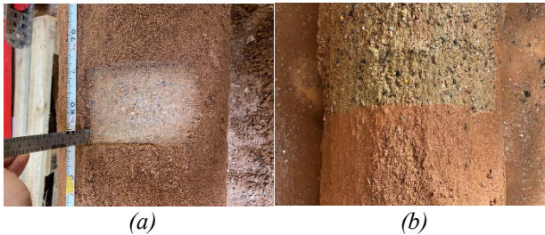
Figure 7. Pile-soil interface observed after exhumation of, (a) bentonite pile, (b) polymer pile
