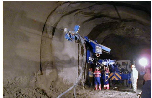
Figure 3. Installation setup for the Gotthard Base Tunnel Safety doors
