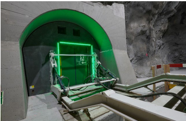
Figure 3. Installation setup for the Gotthard Base Tunnel Safety doors
