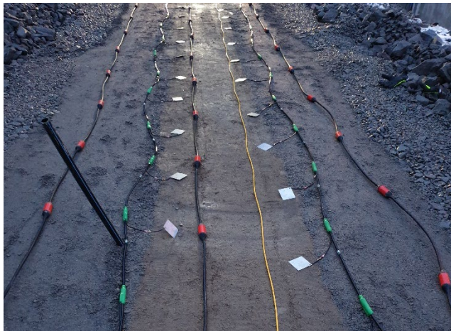
Figure 4. Fibre optic cable (yellow), ERT cables (green/silver) and hydrophone cables (red) at the crest of the core soil before being covered with fine filter and shell fill.
