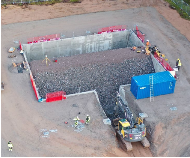
Figure 1. Overview of the concrete containment box and test embankment dam prior to the installation of an uninsulated tent.
