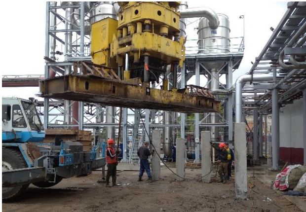
Figure 1. Crane-assisted placement of the piling machine
