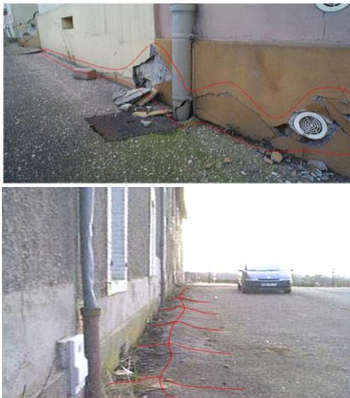
Figure 3. Example of serious structure damages due to subsidence – Iron mine – Lorraine – France.
