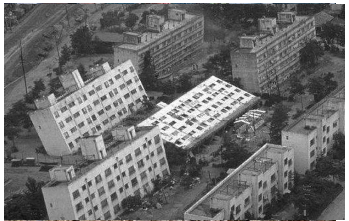
Figure 1. Effects of earthquake-induced liquefaction during 1964's Niigata Earthquake (Penzien, 1964).
