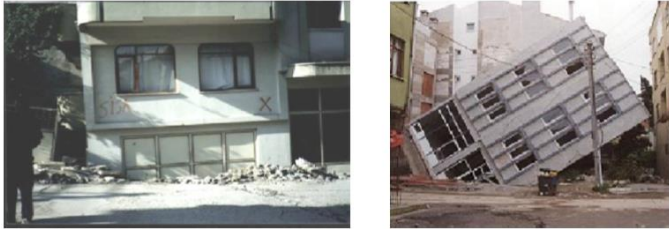
Figure 2. Liquefaction induced damage during the Kocaeli earthquake of 1999 in Turkey (adapted from Madabhushi and Haigh, 2009).
