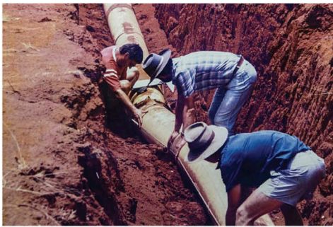
Figure 1. Failure of an API.5L X60 steel gas pipe during the 1999 Tennant Creek, Australia earthquake (source: Geosciences Australia).
