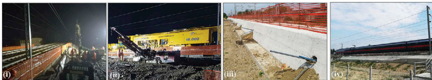
Figure 6. Advancement work for the embankment consolidation with the innovative system.
