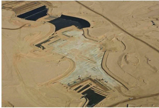
Figure 5. Aerial photo – laid geomembranes partly with concrete covering.
