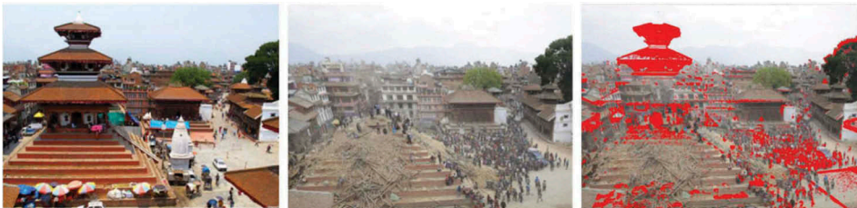
Figure 3. Visual Damage Estimation algorithm result: the difference image (right) shows the detected differences between the original appearance of the building (left) and the post-event image (center).
