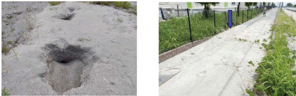
Figure 2. Typical surface manifestation of soil liquefaction at Kumamoto port.
