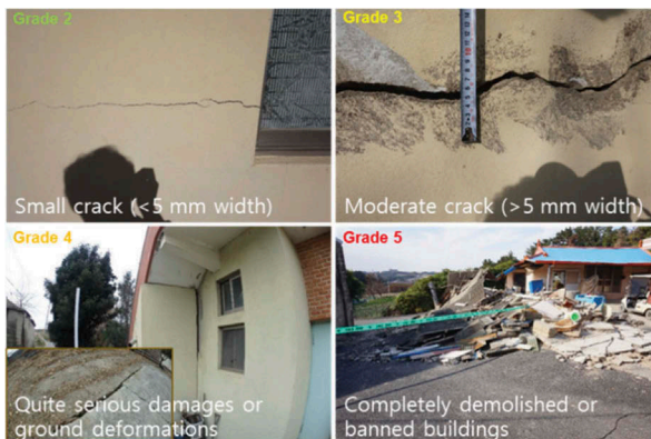
Figure 4. Examples of the criteria used to classify Damage Grade 2 through 5. If no damage is observed, Damage Grade is classified as 1.
