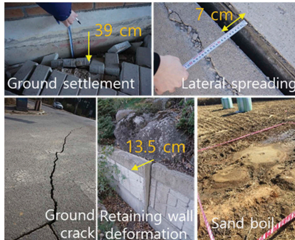
Figure 2. Examples of ground deformations caused by the 2017 Pohang earthquake.
