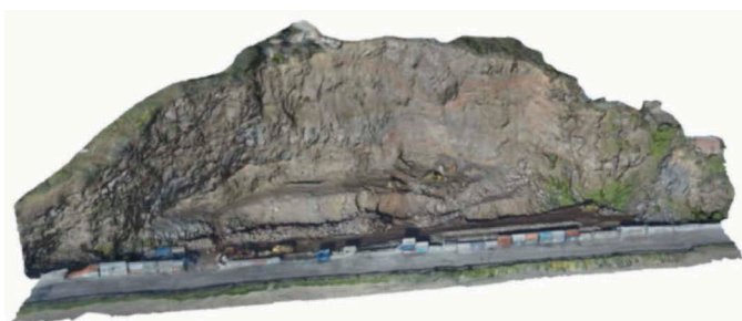
Figure 6. 3D photogrammetry model of the Shag Rock Reserve showing talus debris removal works.
