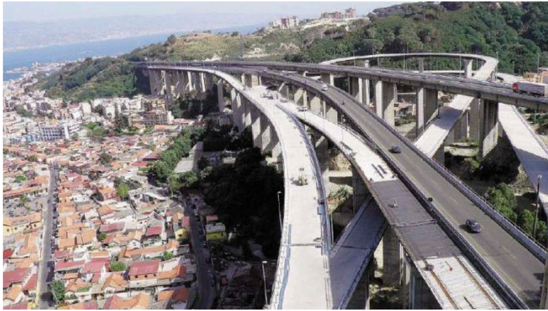
Figure 1. Viadotto Ritiro along motorway A20.
