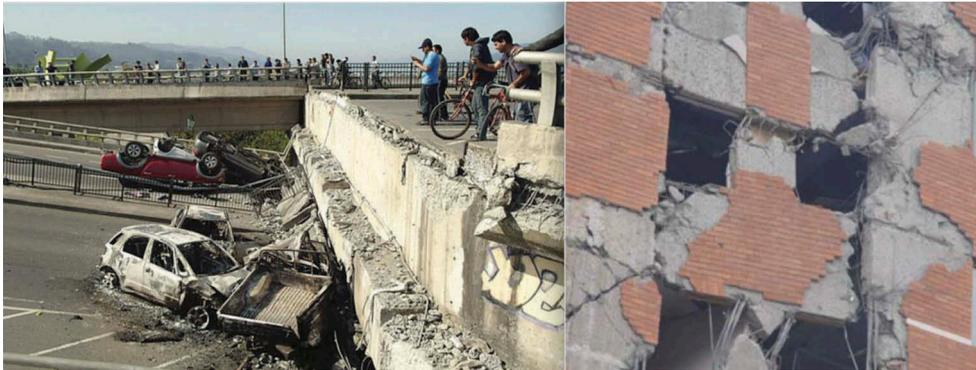
Figure 8. Collapsed bridge in Concepcion shown on the left and damaged apartment building on the right.
