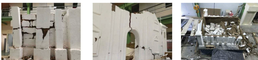
Figure 9. Damage to the Church of San Raymundo
