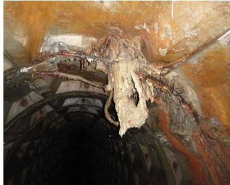
Figure 5. Damage of the protective layer of concrete and tubing armature in the DG central part.
