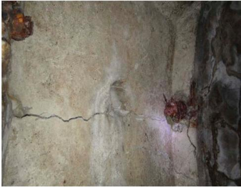
Figure 4. Crack in the concrete of the DG armature upper tubing.
