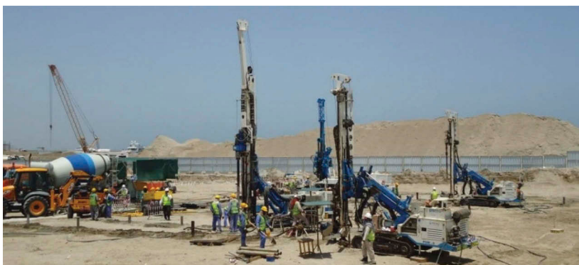
Figure 9. General view of the jobsite and compaction grouting equipment in action.
