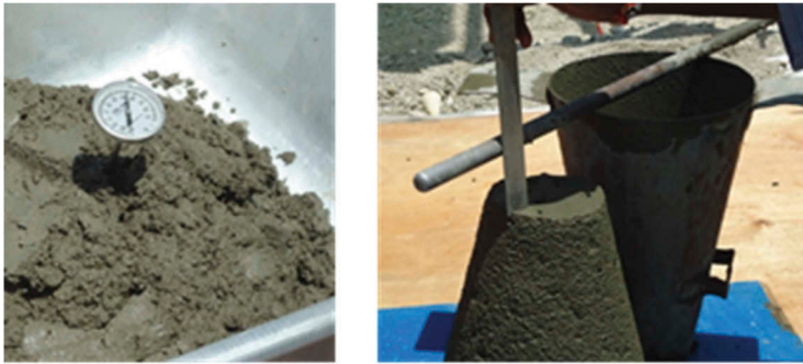
Figure 10. Routine quality controls on the ready-mix mortar delivered at site.
