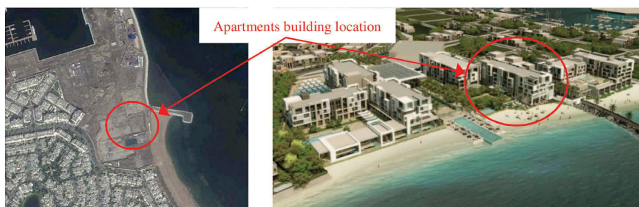
Figure 2. Aerial view and render of the new Kempinski Hotel and Apartments complex at “The Wave”.
