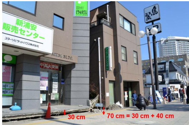
Figure 1. Observed Liquefaction-Induced Settlements after 2011 Tohoku Earthquake (Ashford et al. 2011, Bray 2016).
