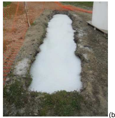
Figure 6. Photos of barriers: (a) inverted pyramid barrier and (b) linear barrier.
