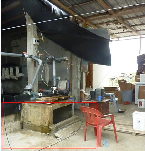
Figure 2: Relative uplift of structure with underground storage tanks at Pedernales shrimp farm.
