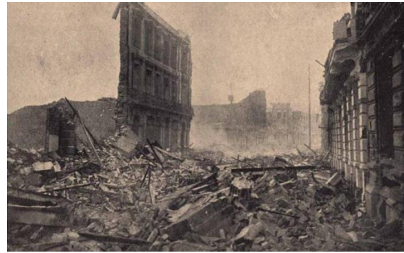
Figure 6. Total destruction in the area of ground consisting of a sandy soil deposit (intersection of Blanco and Edwards streets).
