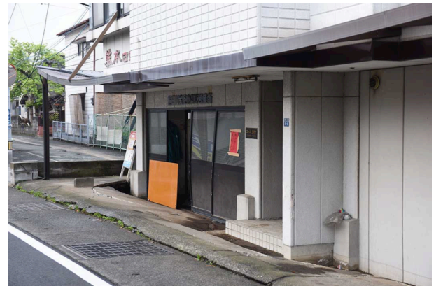
Figure 3. Liquefaction-induced settlement of a 3-story reinforced concrete building in Karikusa town
