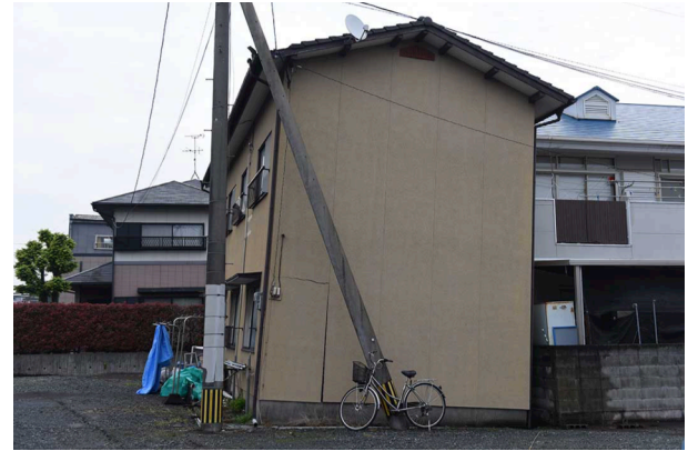
Figure 2. Liquefaction-induced tilt of a 2-story wooden house in Karikusa town
