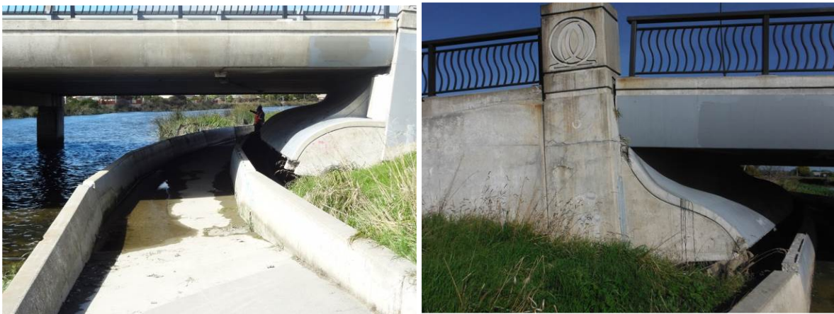
Figure 4 Rotation of south abutment from west (left) and east (right)
