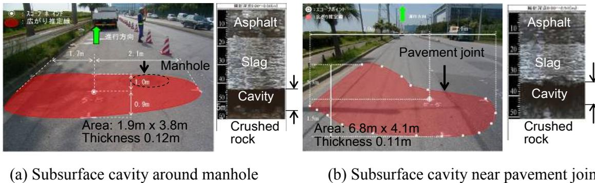
Figure 2. Examples of liquefaction cavities.
