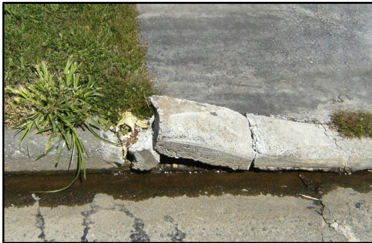
Figure 5: Kerbing in Roscoe Street. Such evidence of lateral compression was observed in kerbing at many sites in east-west oriented streets in the Hillsborough Valley floor.
