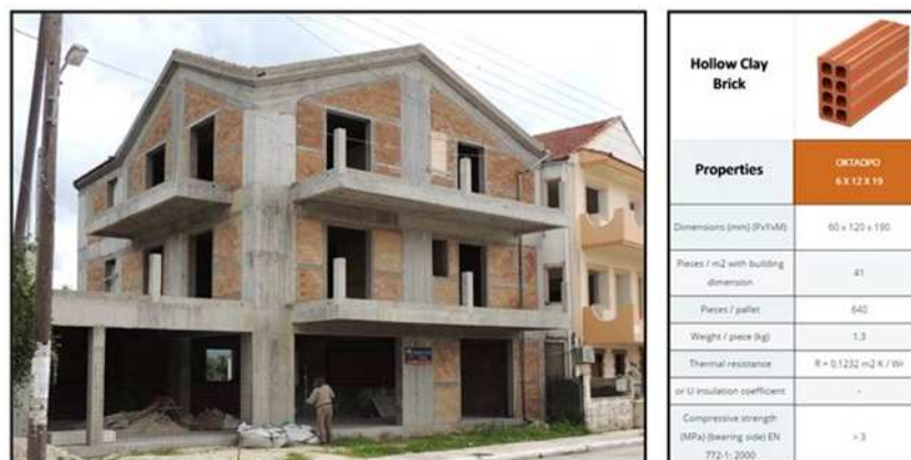
Figure 7. Confined masonry construction (left); properties of infill clay bricks (right).
