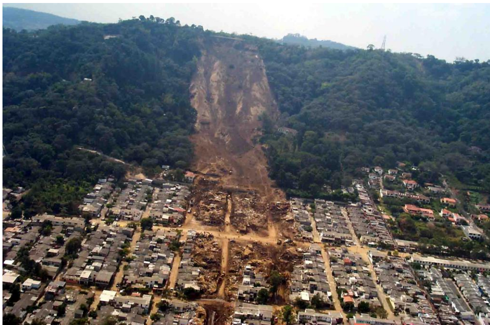
Figure 1. Las Colinas Landslide (Crosta et al., 2005)
