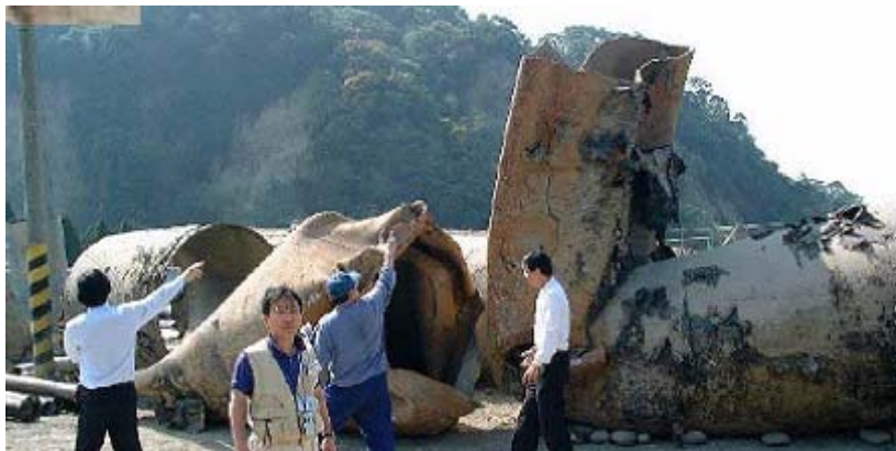
Figure 2. An example of damaged pipeline due to faulting
