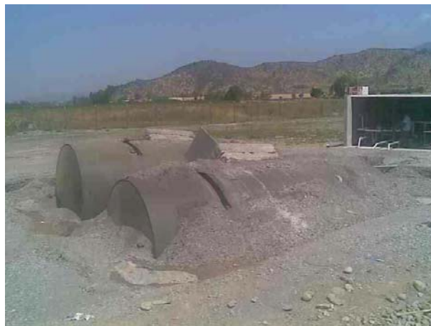
Figure 1. Tanks buoyed above the ground surface during the 2010 Chile earthquake (GEER, 2010)
