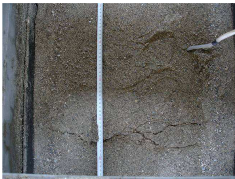
Fig. 7. Tensile cracks observed in sand backfill
