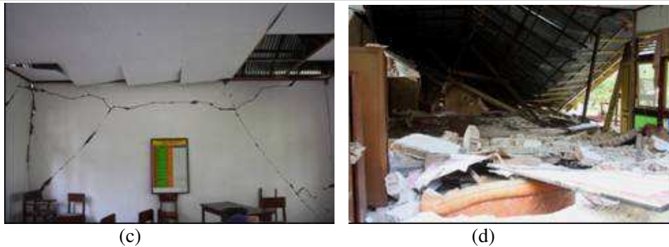
Figure 3. Typical damage on unreinforced masonry residential house and school in Pariaman, Padang Pariaman and Agam district.
