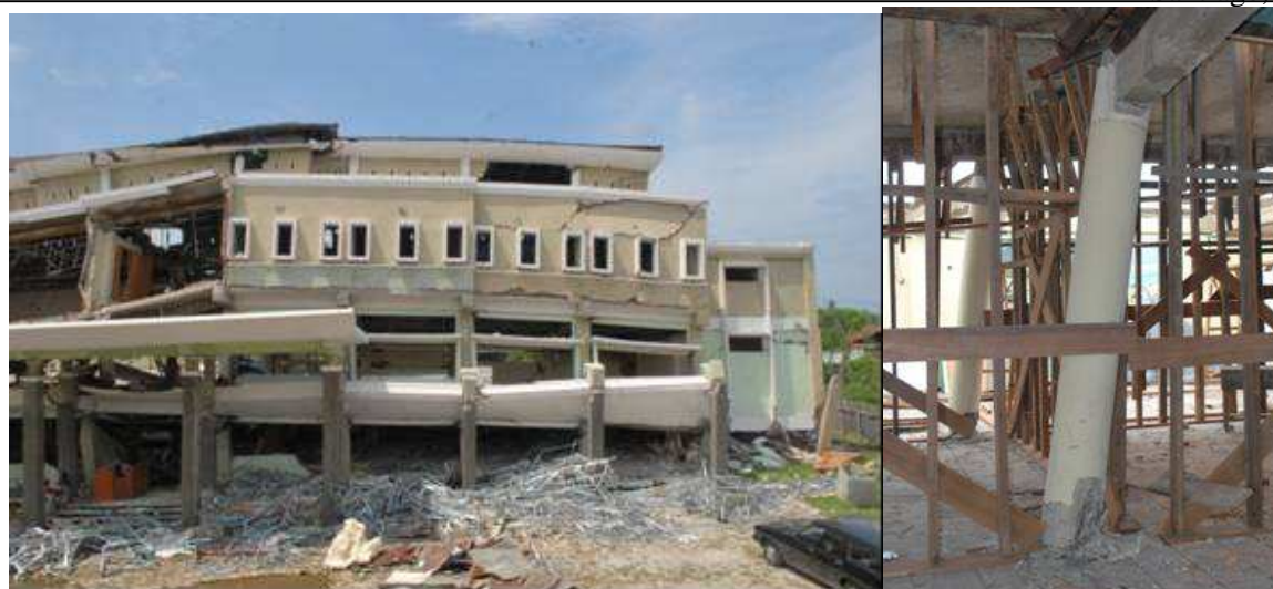
(a) (b) Figure 7. Severe damage on reinforce concrete buildings in Padang city due to poor column detailing
