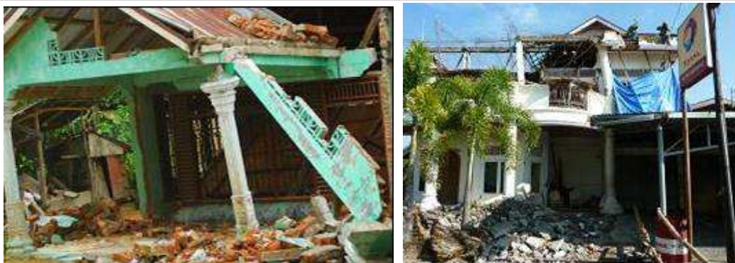
Figure 5. Collapsed and severe damage masonry building with simple reinforced concrete frame system in Padang Pariaman and Padang city district due to low quality of building design or material
