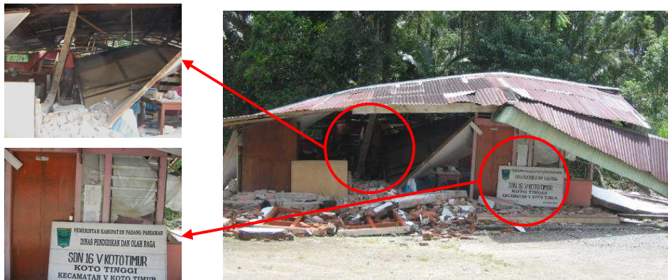
Figure 4. Collapsed school building in Koto Tinggi, Padang Pariaman district due to walls which tend to separate from the supporting foundation
