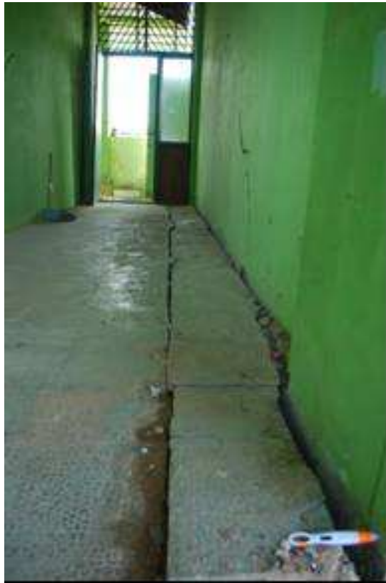
Figure 9. Typical damage on buildings due to soil settlement
