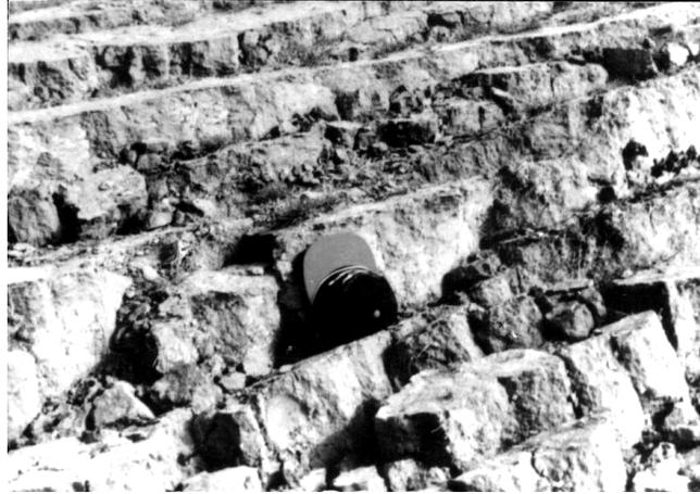
**Figure 1. The step-like fissure caused by seismic settlement (by J.S. Liu, 1995)**
