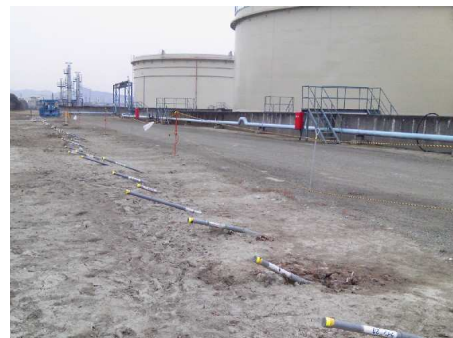
(b) Installed grouting pipes
