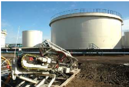
(a) Directional drilling towards ground beneath tank
