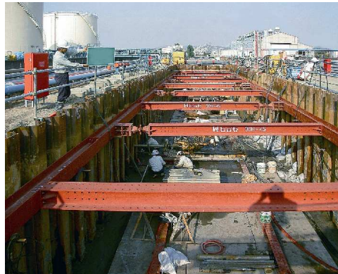
Figure 2. Conventional horizontal grouting from a vertical shaft
