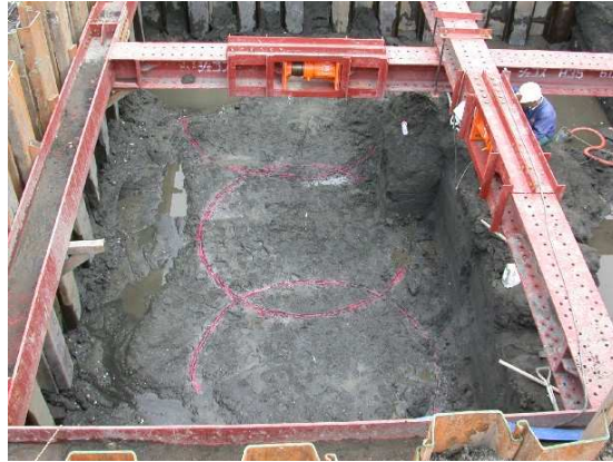
Figure 7. Exposed solidified ground sliced at GL-2.5m
