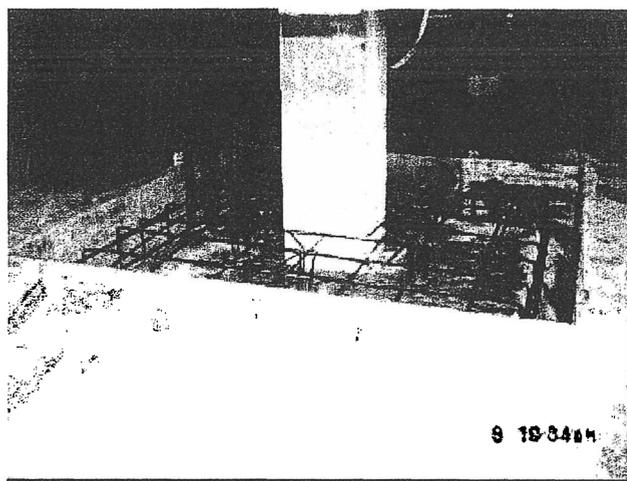
Fig. 2 Reinforcement of footings
