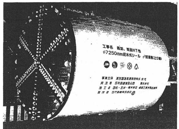
Figure 3 General view of Slurry shield machine
