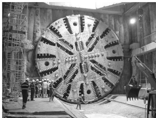
Figure 5. 12 m diameter EPB machine.
