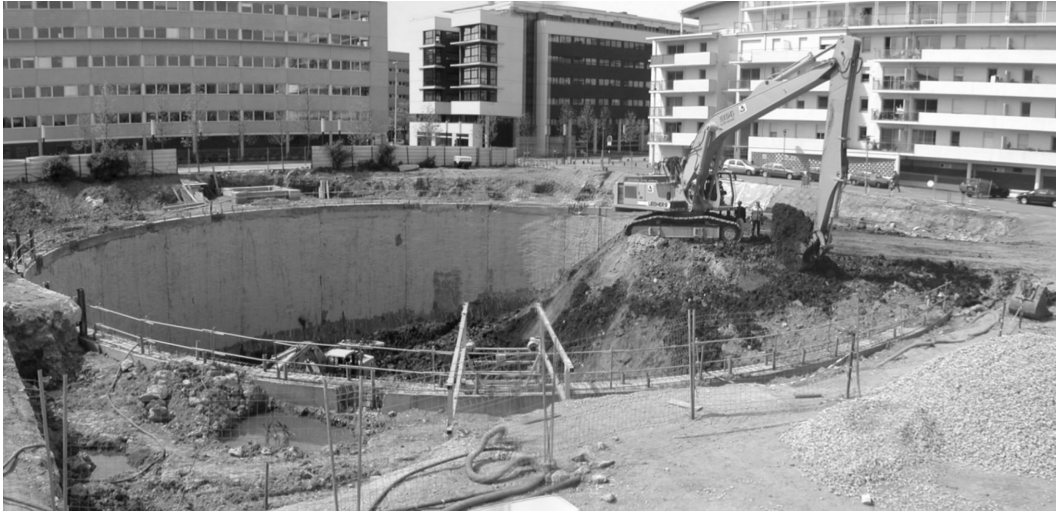
Figure 2. Dissymmetric soil excavation inside the diaphragm wall. Solétanche-Bachy, 2002.
