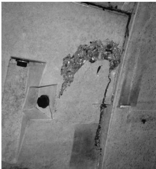
Figure 2. Damage to the Dowel and notch sockets.
