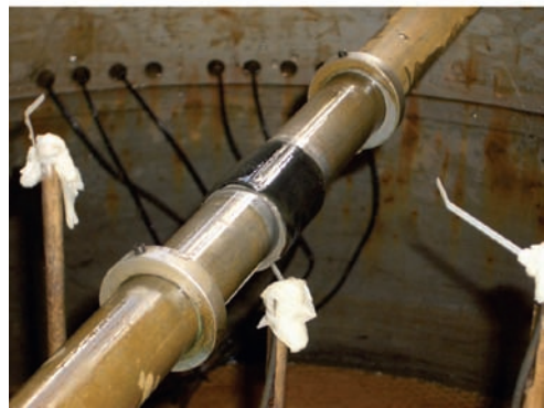
Figure 4. Simplified model of Tube à Manchette (TAM) used for injection. Actual space between the two rings is 40 mm during injection (Bezuijen et al. 2007).
