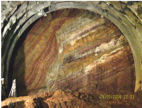
Figure 2. A South Toulon tunnel face.
