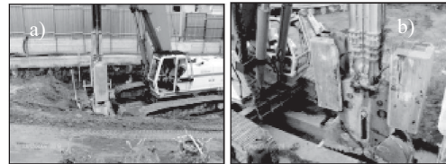
Figure 7. Pictures from the site in Napoli: different positions of the operating machine during panel excavation: a) on the long side; b) on the short side.
