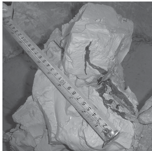
Figure 3. Grout injection in silt.
