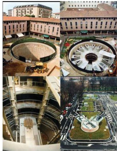
Figure 1. TreviPark construction sequence: secant piles retaining wall and excavation, placing of prefabricated internal structures, installation of car lift and final urban facilities.
