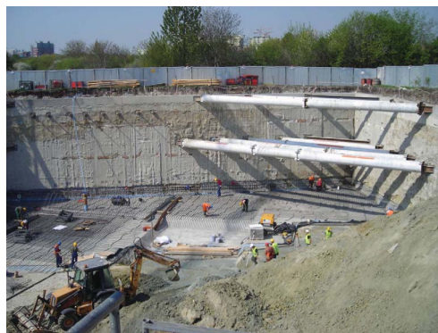
Figure 1. Construction site “Canal+”.
