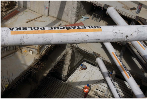
Figure 4. Construction site at Prosta St.
