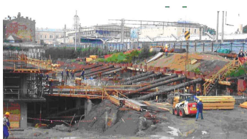
Figure 11. View of struts in the ditch.
