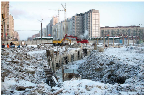
Figure 2. Initial trench made by “Wall in ground” method (a) and sheet pile immersion (b).
