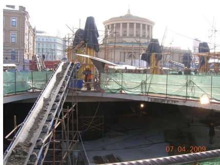
Figure 9. Excavation of the soil under the ceiling.
