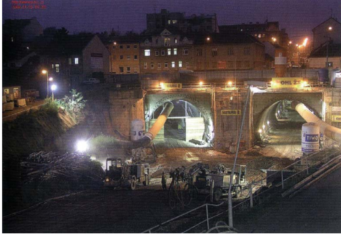
Figure 1. Temporary portals of the Kralovo Pole tunnels (Horák 2009).
