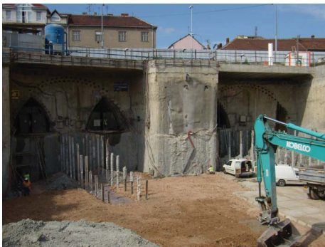
Figure 3. Exploratory drifts situated in the top headings of the future Královo Pole tunnels.
